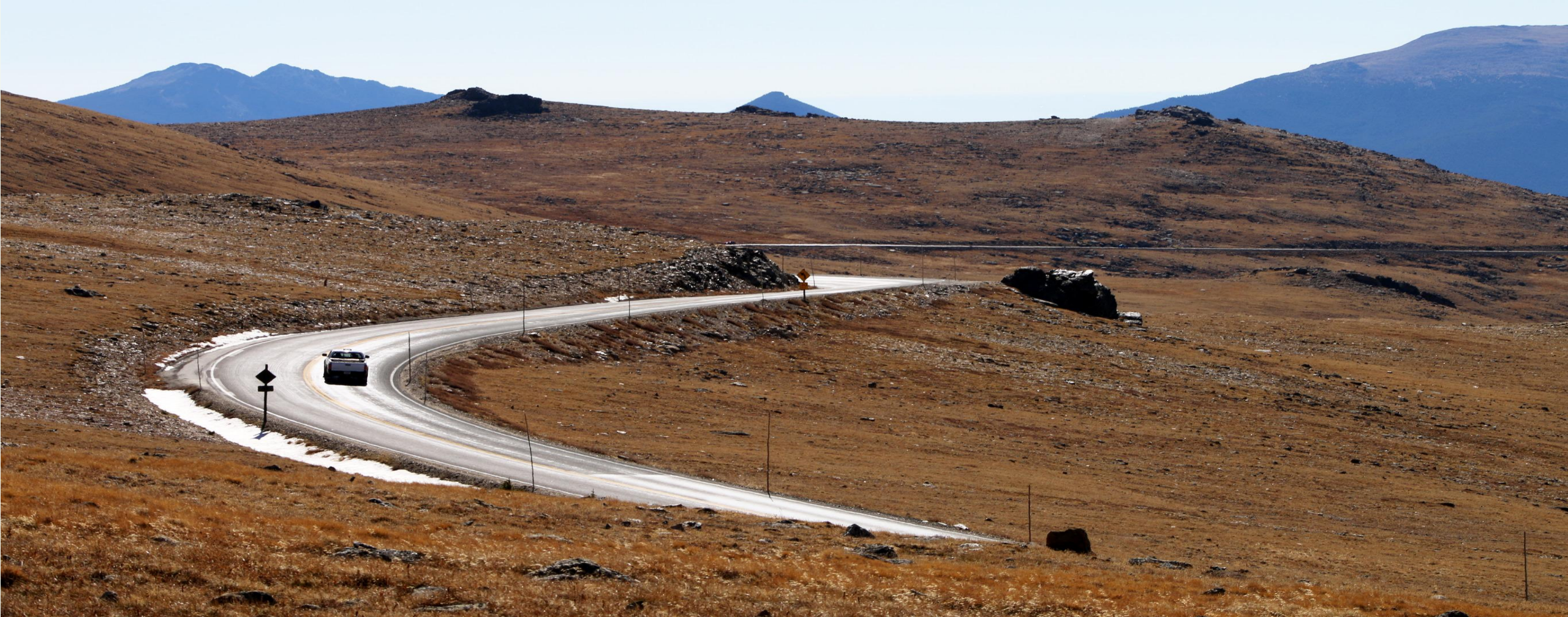
Visitors drive along Trailridge Road in Rocky Mountain National Park NPS/M.Reed
